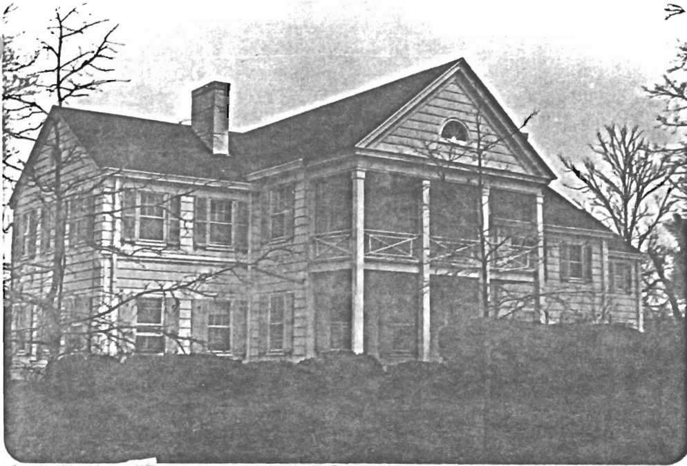
House (E) View Northeast
