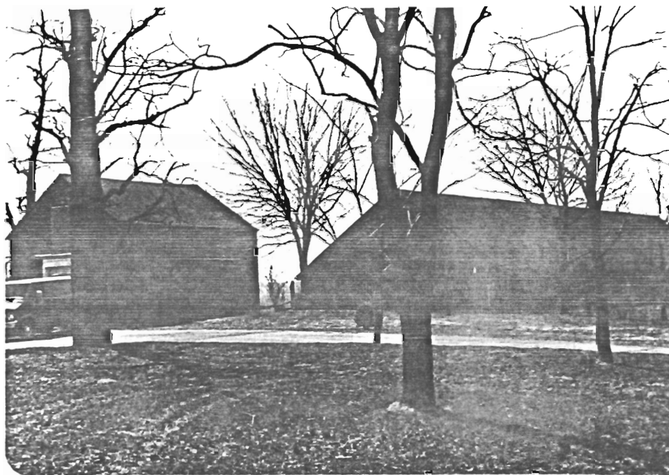
Barns; facing S.W.
